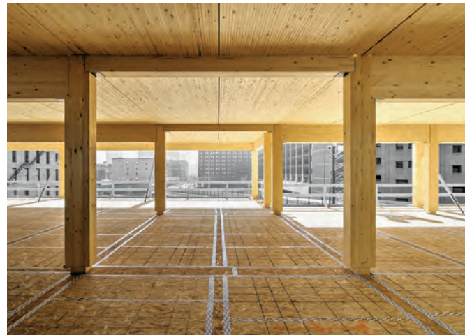
FIGURE 2-5: NLT decking in the seven-story T3 Minneapolis Image: MGA | Michael Green Architecture, Ema Peter
