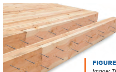
FIGURE 2-5: NLT decking in the seven-story T3 Minneapolis Image: MGA | Michael Green Architecture, Ema Peter
