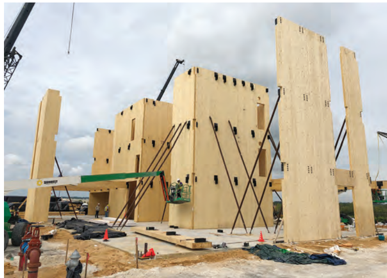
FIGURE 5-50: Don't remove bracing without approval from the EOR
