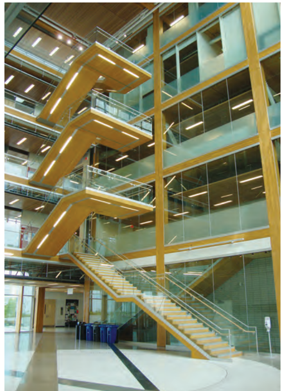
FIGURE 5-49: Examples of feature stairs at Albina Yard (top) and the Earth Sciences Building at the University of British Columbia
