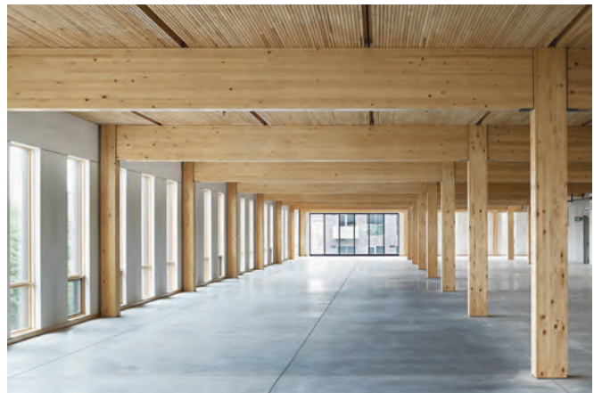
FIGURE 2-12: Glulam post-and-beam framing supports DLT at 111 East Grand in Des Moines, IA Image: Neumann Monson Architects, photo Mike Sinclair
