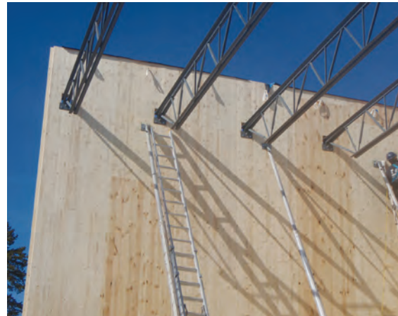
FIGURE 5-29: Roof with open-web steel joists supported by CLT walls Images: Moses Structural Engineers, Inc.
