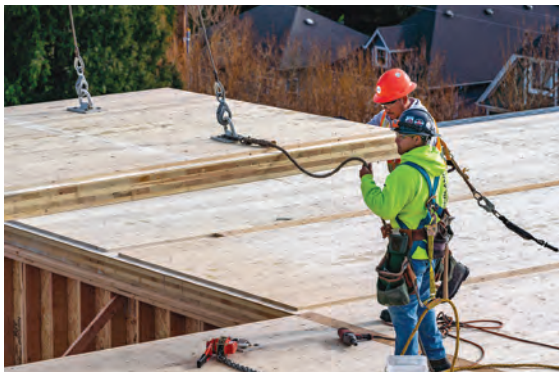
FIGURE 5-2: Hoisting anchors on CLT panels at The Canyons in Portland, OR
