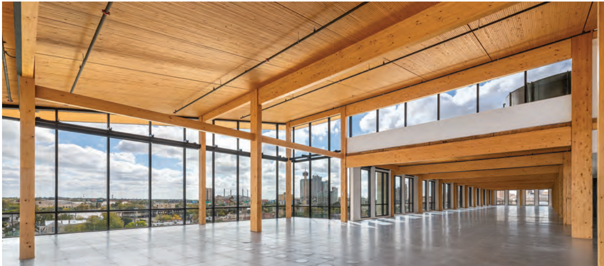
FIGURE 2-7: DLT decking in The Soto, a six-story office building by Hixon Properties
