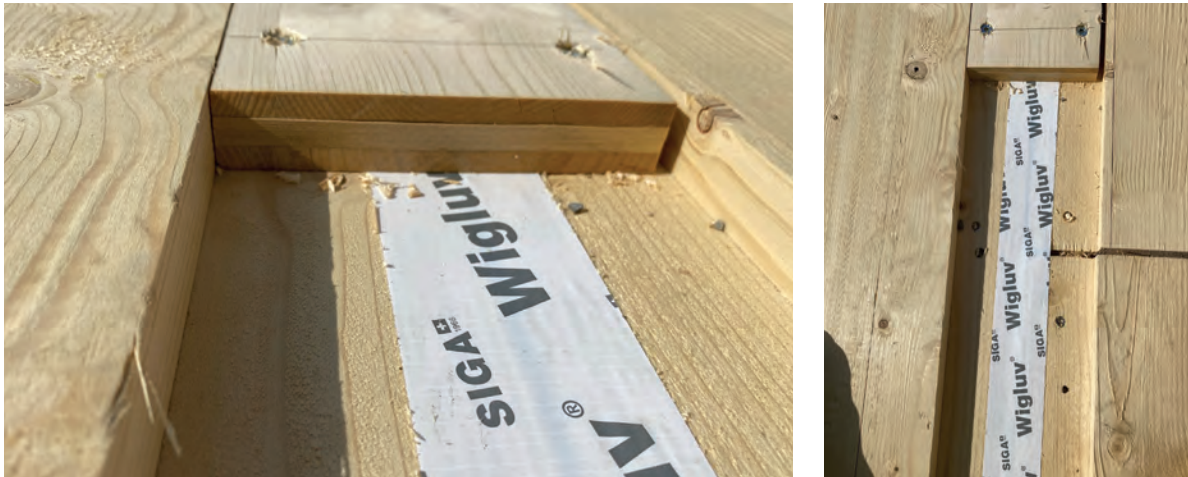
FIGURE 4-6: Panel-to-panel joint taped prior to placement of spline; the spline will be taped after installation.
