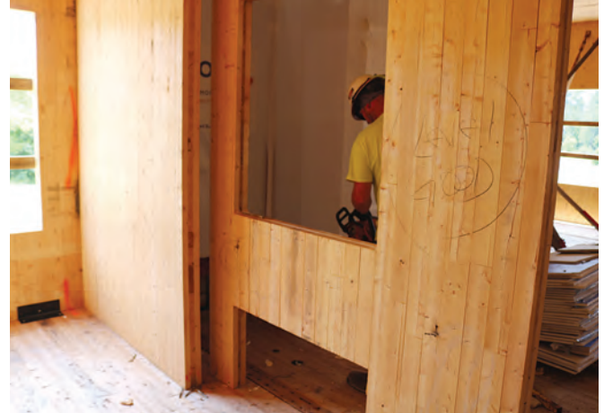
FIGURE 3-8: Partially cut door opening
