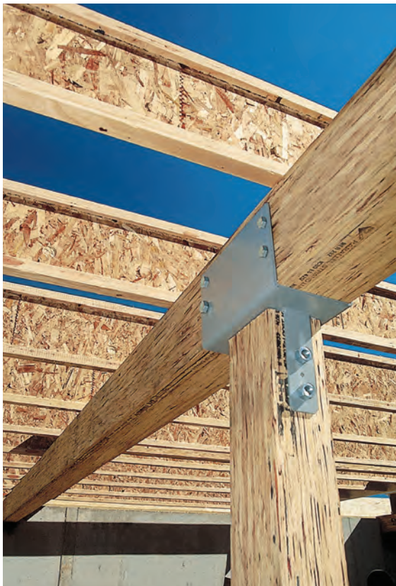
FIGURE 2-11: PSL beams Image: Weyerhaeuser
