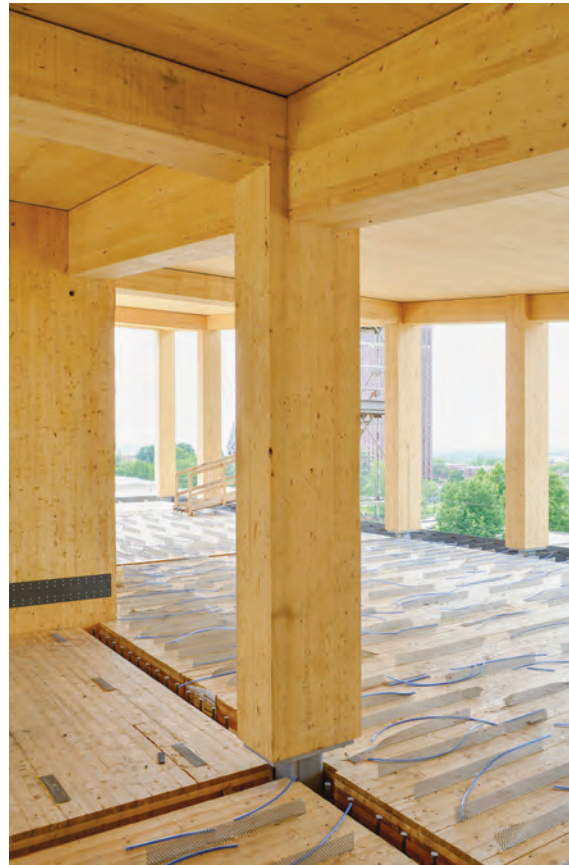
FIGURE 2-14: CLT-concrete composite floor system at the John W. Olver Design Building at UMass Amherst
