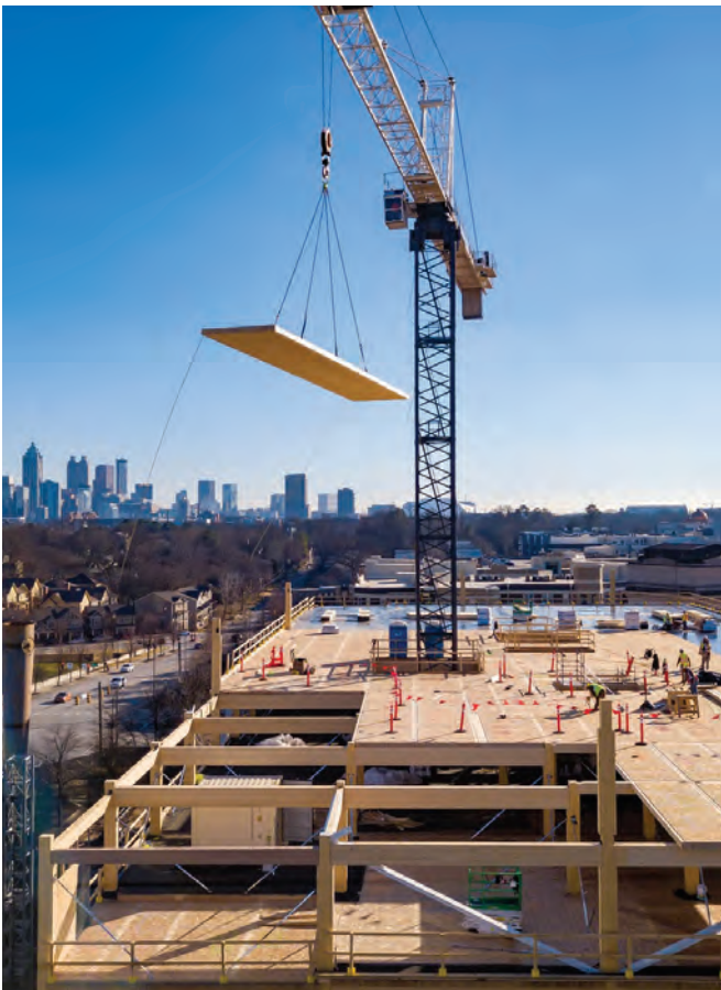
FIGURE 5-1: Tower crane positioned for access at T3 in Atlanta, GA
