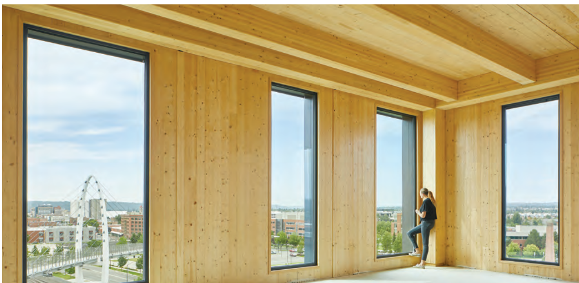
FIGURE 2-2: CLT walls and ceiling in the five-story Catalyst in Spokane, WA
