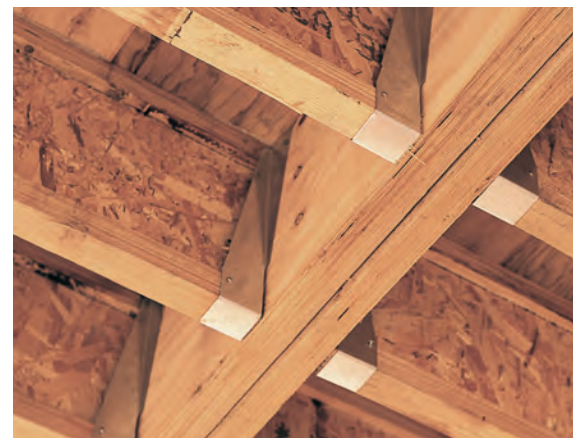
FIGURE 2-9: LVL beams
