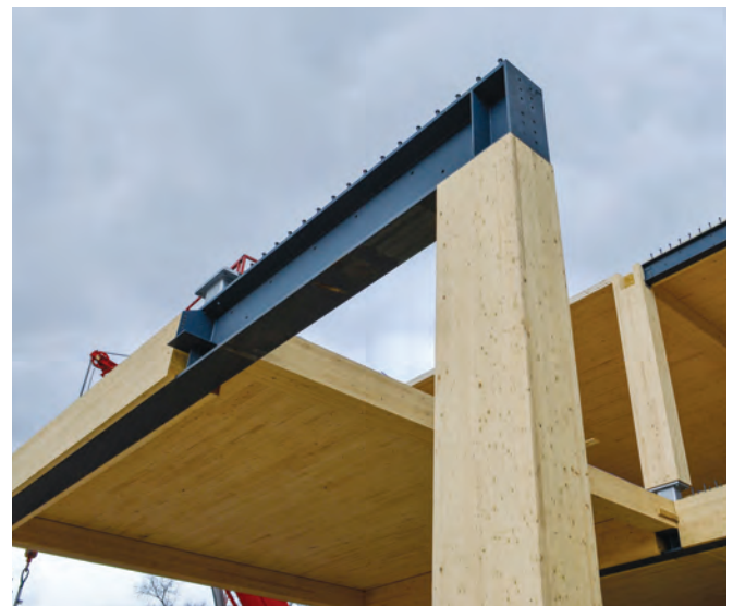
FIGURE 5-28: Steel beams bearing on timber columns Images: Alex Schreyer
