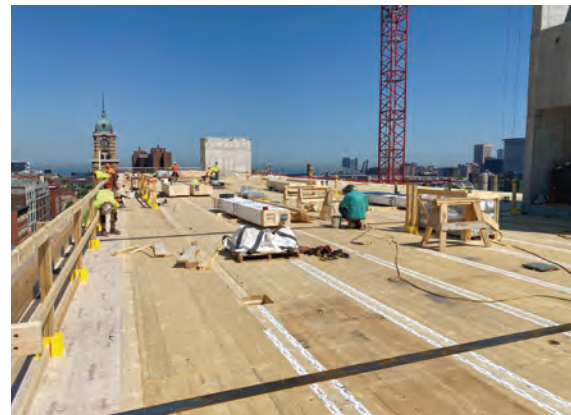
FIGURE 4-7: Upper level with completed spline/tape and in-process areas
