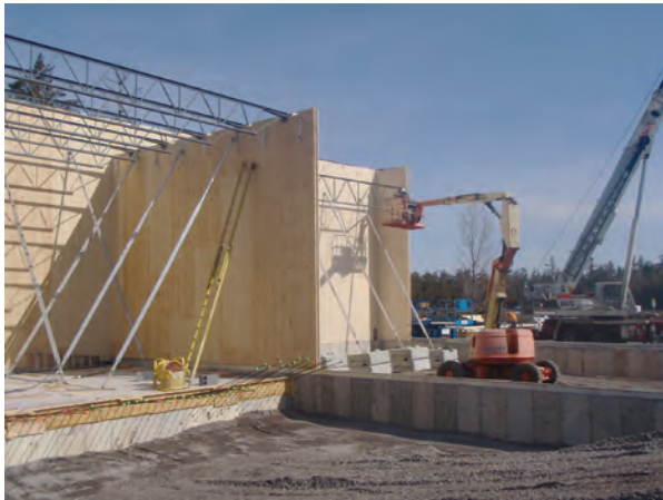
FIGURE 5-29: Roof with open-web steel joists supported by CLT walls Images: Moses Structural Engineers, Inc.
