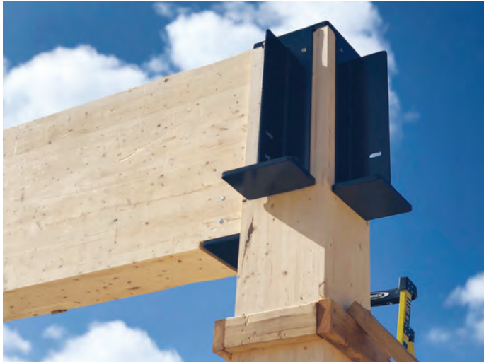
FIGURE 5-20: Beam-to-beam-to-column corner connection
