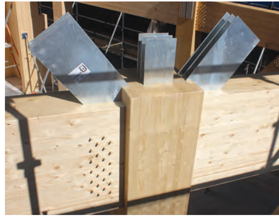
FIGURE 5-21: Concealed metal plate connections
