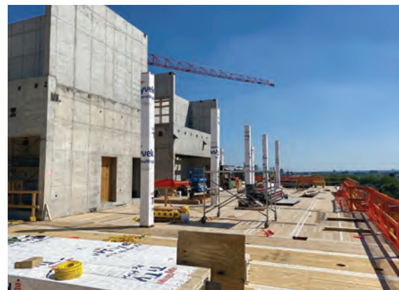
FIGURE 4-8: Fully taped/installed spline
