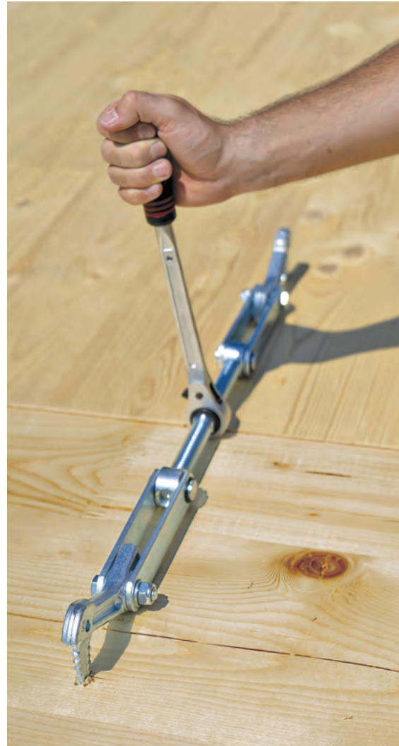
FIGURE 5-45: Tight fit between panels is ensured using special installation devices, though it's important to maintain required gaps Images: Rothoblaas
