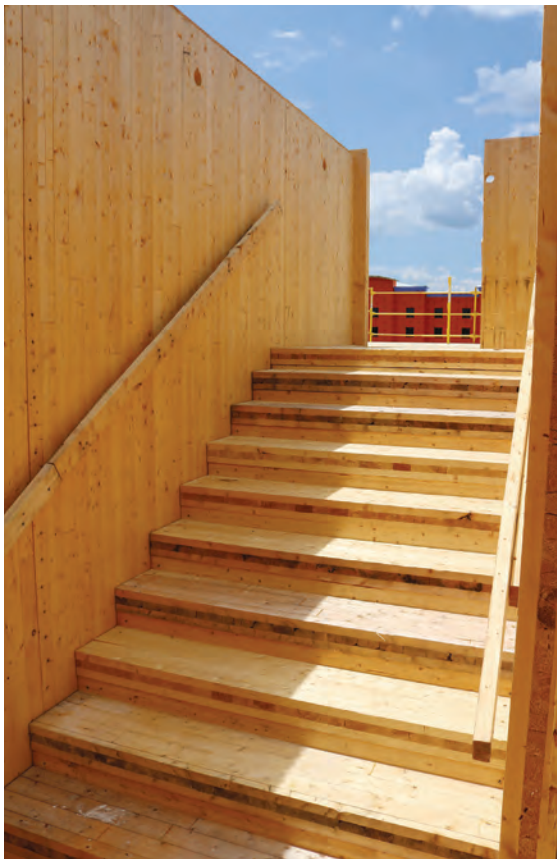
FIGURE 5-48: Example of egress stair
