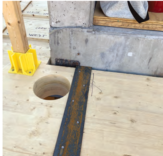
FIGURE 5-7: Gap between wood floor and concrete core allows for different tolerances Image: Anthony Harvey, WoodWorks
